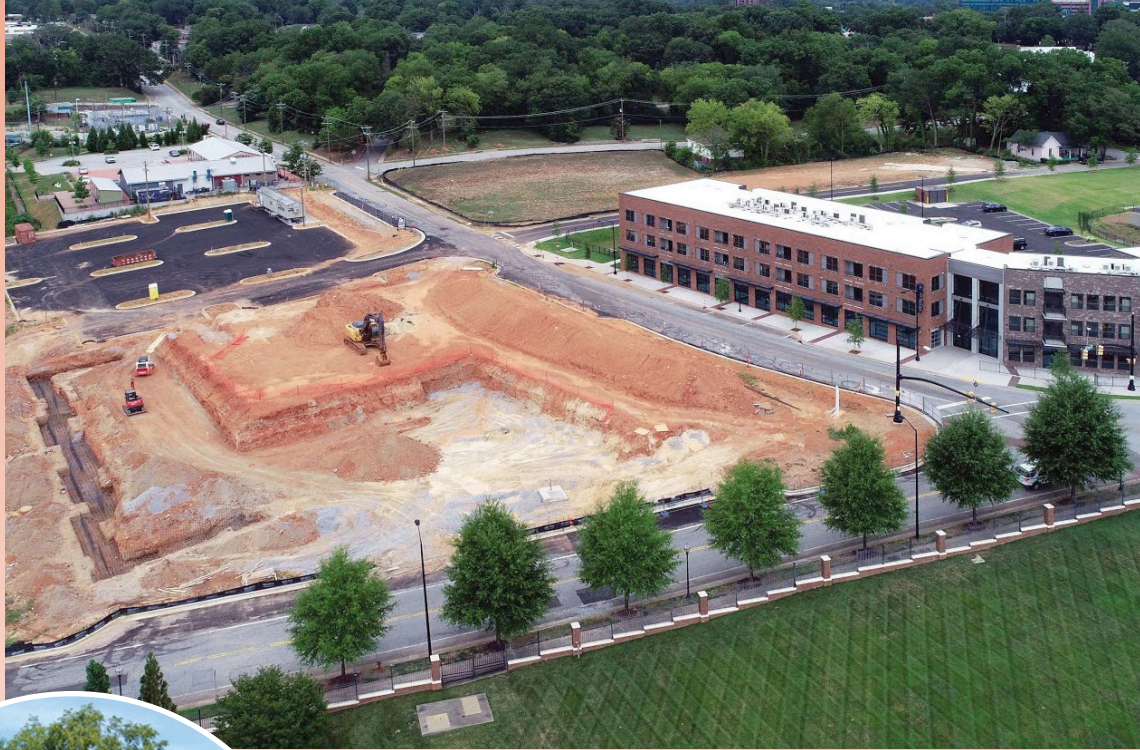
Northside Station Construction
